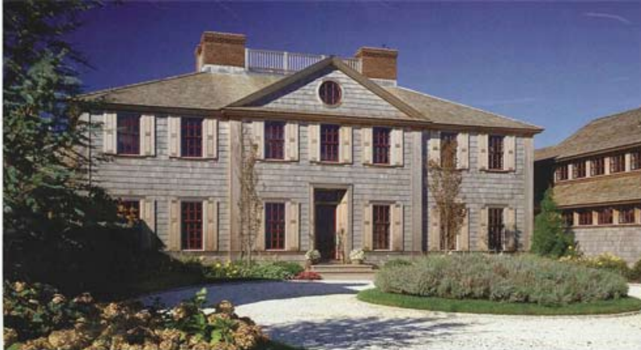
A circular drive of crushed white shells leads to the main section of Sand Dollars, which features eight-in.-exposure Alaskan yellow cedar shingles, a red-cedar shingle roof and deep red window sashes and doors. Photo: Brian Vanden Brink
