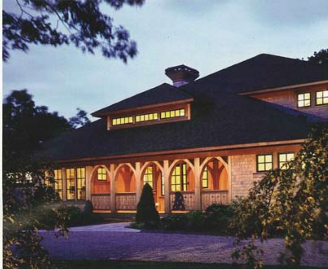
Built as a vacation home for a family with four children, this house, on Lake Wequaquet in Centerville, MA, is reminiscent of Victorian summer cottages and 1920s bungalows. Photo: Randall Perry
