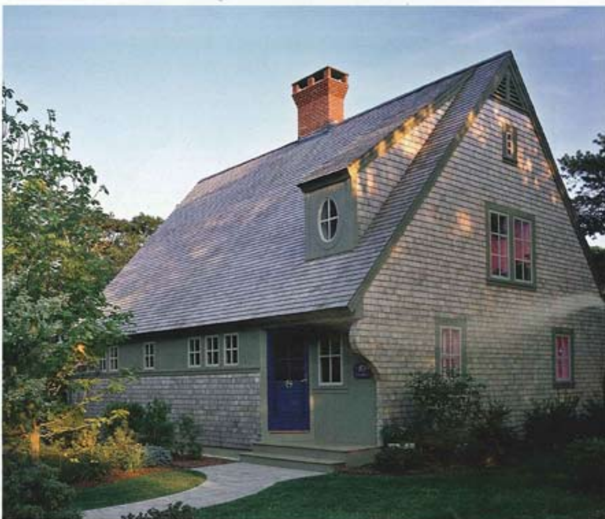
This storybook Cape, a vacation home on Cape Cod, was sited to get the best view of the distant water. Photo: Randall Perry
